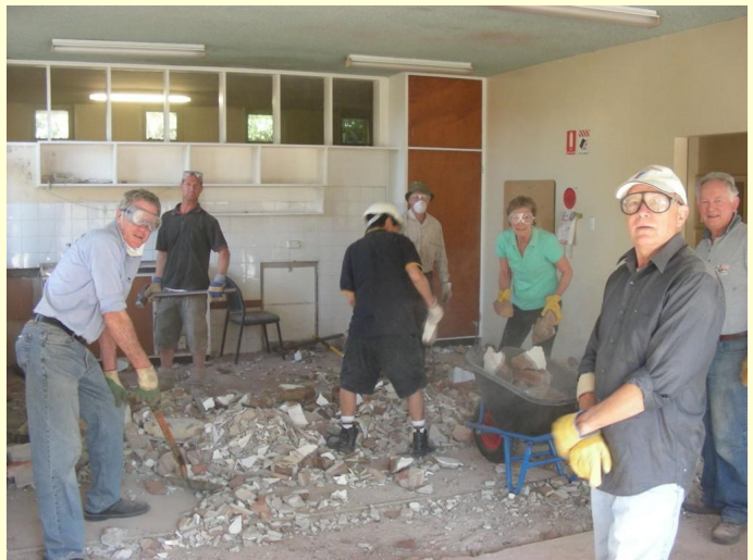
The club's demolition squad in action
